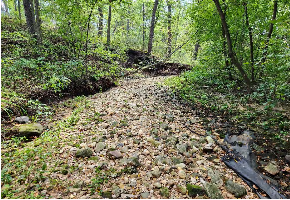
Figure 3. Bank and bluff erosion observed in the armored lower segment of Pennito Creek. Note large bar of mobile bedload and exposed underlying geotextile fabric (photo Inter-Fluve).
